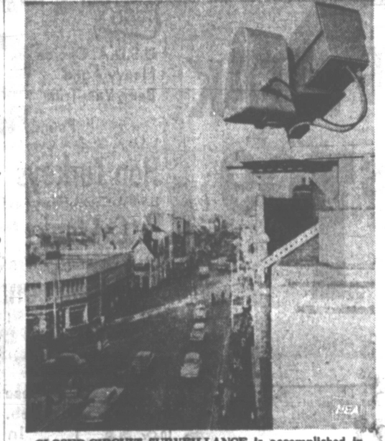
CLOSED-CIRCUIT SURVEILLANCE is accomplished in Croydon, England, with television cameras mounted at strategic positions in the district. Each camera can be rotated 360 degrees by remote control from the central monitoring unit at the police station.
