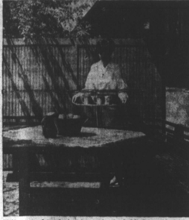
Tall screen of 1x2-inch western pine in 4x4-inch post framing sets off patio for brunches, afternoon snacks. Table top is 2x6-inch Douglas fir laid flat, on 4x4-inch legs. Bench seats are 2x4-inch fir on edge, backrests 2x2-inch fir.
