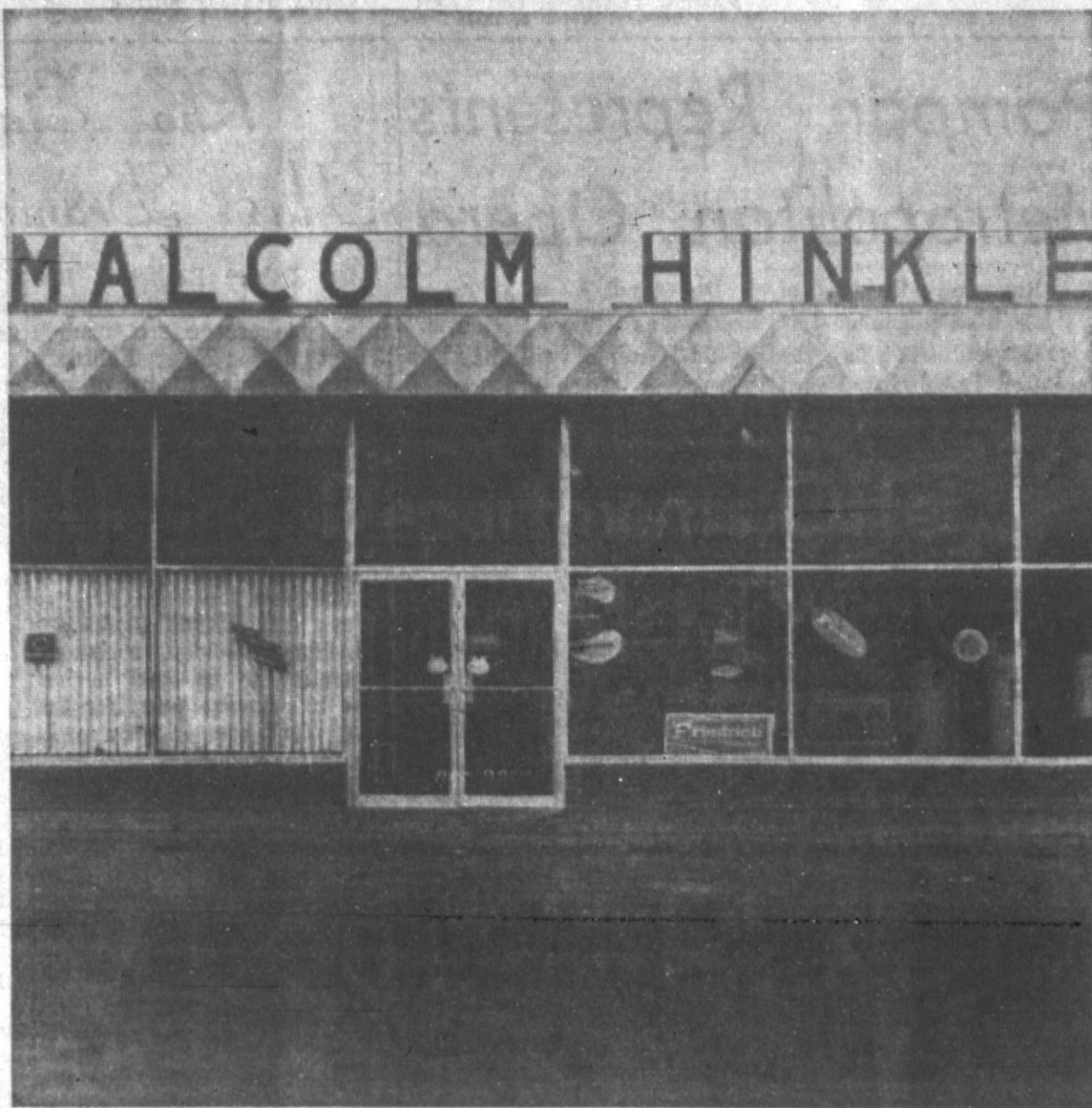
EXPERT SERVICE — Malcolm Hinkle Inc. continues to serve the Pampa trade area and is bonded to operate in five states to assure complete service in the fields of sheet metal, plumbing and heating. (Staff Photo)
