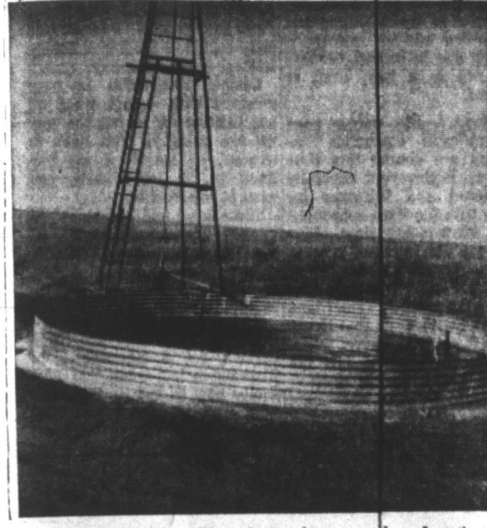
TANK WATER — The photo shows a water storage facility that was constructed with assistance through the Great Plains Conservation Program on the Aaron and Raymond Sullivan farm near MeLean.
