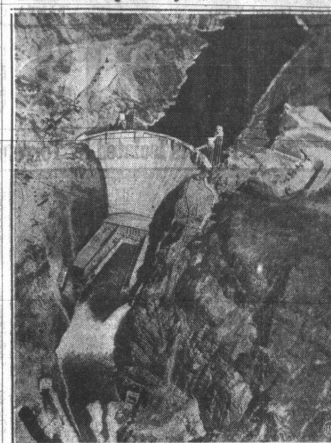
Not a tiny model, but the real, massive Boulder Dam, with great torrents gushing through its spillways for the first time, is pictured in this striking view, taken from a plane high above the earth. Enough water to float a battleship poured from Boulder Lake through the intake towers, shown behind the dam, and out the giant spillways, so government engineers could test the equipment.
