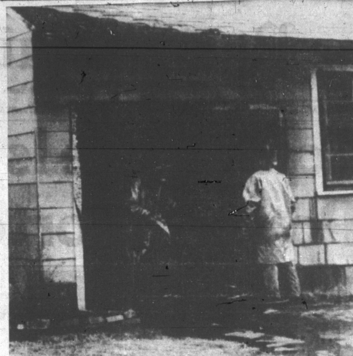
DAMAGED GARAGE — Two Pampa firemen, Tommy Brewer and Carl Mann, help extinguish a garage fire at the home of Bobby Shoopman, 1021 S. Wells, which caused heavy damage to the garage, but no injuries. Firemen said an open face heater caught gasoline on fire while Shoopman was working on a carburetor in the garage. The garage is owned by Royce Logan of Corpus Christi. (Staff Photo)
