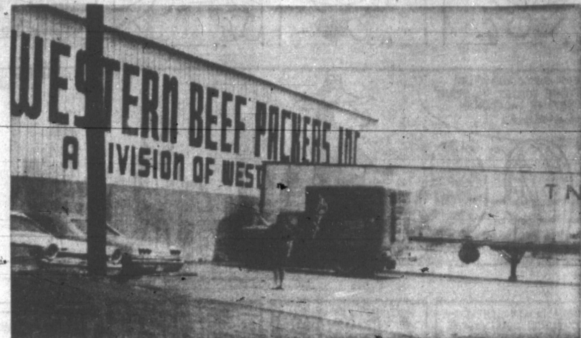
WESTERN BEEF PACKERS INC. — Western Beef Packers is a member of the ranks of newer businesses in Pampa. All extensive updating and expansion of the facilities was completed in 1970 making it one of the most modern meat processing plants in the area. It has helped promote agri-business success here, and continues to grow. (Staff Photo)
