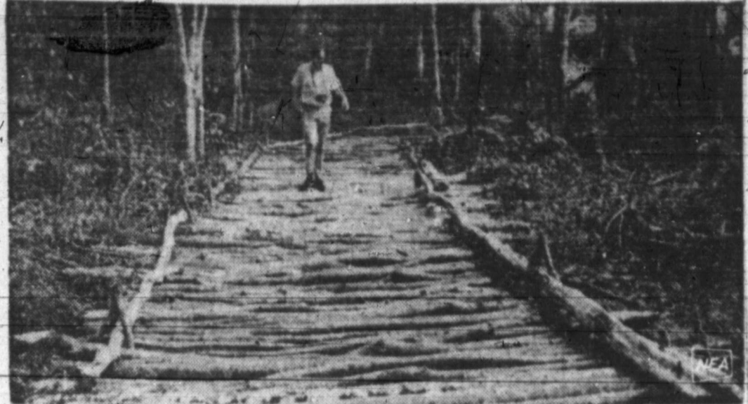
NOT MUCH OF A HIGHWAY, but the corduroy road of tree trunks located near the South Vietnam border on a visit to Cambodia by Ray F. Herndon on a visit to Cambodia plays a vital role in Viet Cong strategy. Discovery of the road, capable of moving heavy supplies into Vietnam, and a deserted guerrilla camp under Viet Cong control denials that its territory served as a Viet Cong sanctuary.
