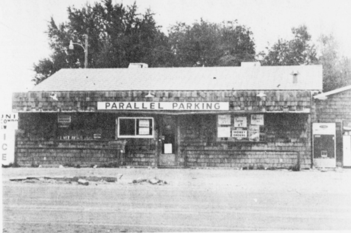
OLD LOCATION 414 West American Blvd.
