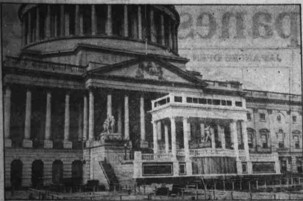
The stand in front of the national capital where Mr. Roosevelt will take the oath as President is nearly completed. (Associated Press Photo)
