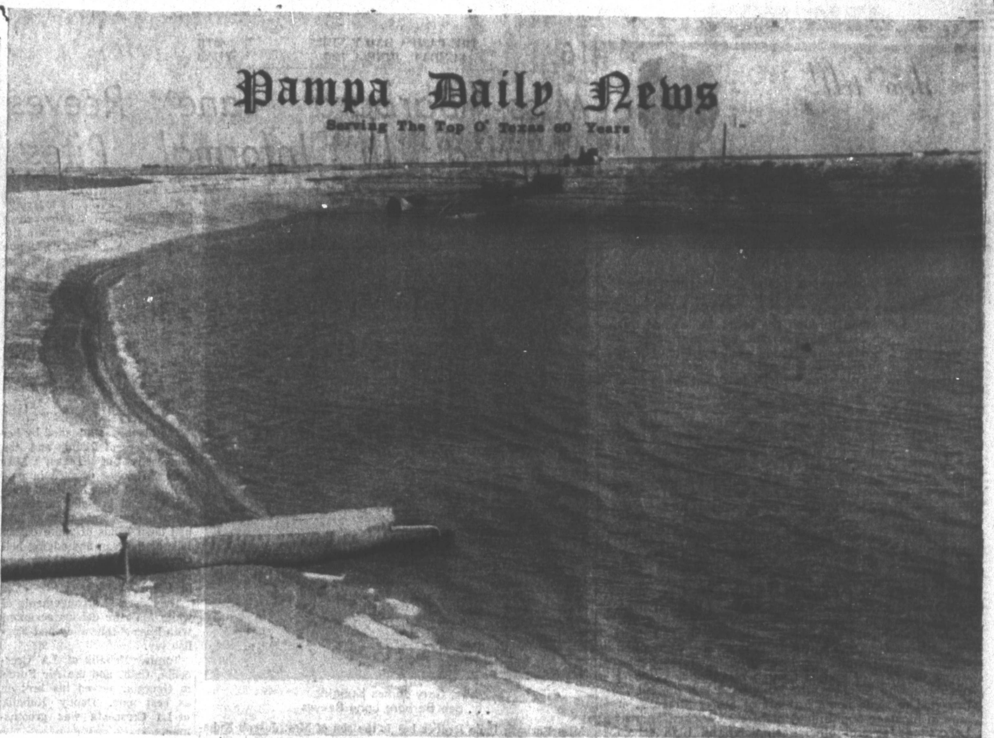
TOMMY ANDERWALD'S TAILWATER RECOVERY PIT IRRIGATES THIRD WHEAT CROP connecting settling basin filters out mud and silt before water flows into pit
