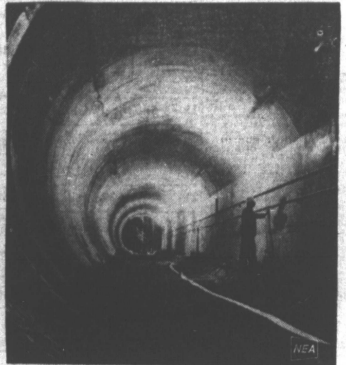
WORLD'S LONGEST underwater tube is beginning to take form under San Francisco Bay. The first of a planned 57 massive steel and concrete sections, such as pictured above, have been lowered into position in a dredged trench near the Oakland shoreline. When completed, the rapid transit tube will stretch four miles between Oakland and San Francisco.
