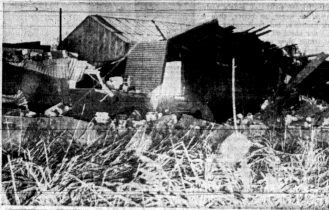
DAMAGED TRUCKS ..in Lee Building
