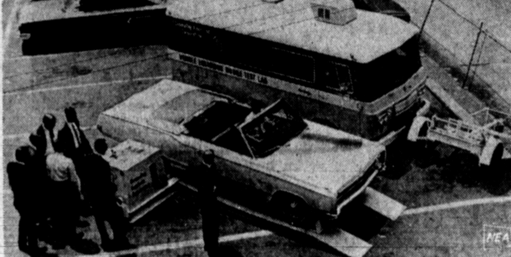
NOT A WASHER, BUT A WATCHDOG is the mobile test station, above, for measuring automobile emissions. Such stations will be needed for surveillance of in-service performance of exhaust control devices, as shown top center, required by federal law on all new cars starting with 1968 models. Top left is a machine that washes dirt from the air by means of water squirting from pinjets. At left is a unit that draws acid fumes through ducts and scrubs them in a water and caustic solution combination.
