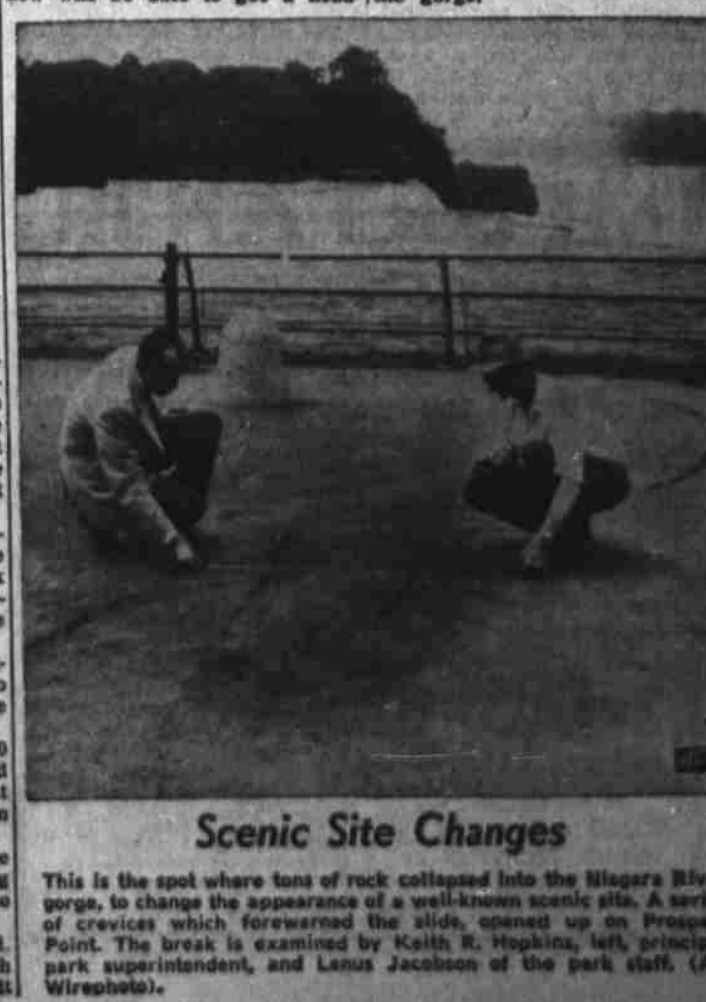
This is the spot where tons of rock collapsed into the Niagara River gorge, to change the appearance of a well-known scenic site. A series of crevices which formed the site, opened up on Prospect Point. The break is examined by Keith E. Hopkins, left, principal park superintendent, and Lenus Jacobson of the park staff. (AP Wirephoto).
