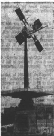
A WINDMILL in Cali-fornia? Actually it's a spacecraft—a test model of spacecraft—a test model of the Venus Mariner sched-uled for launch in June, and currently undergoing tests of its solar panels at the jet propulsion labora-tory of California Institute of Technology near Pasa-
