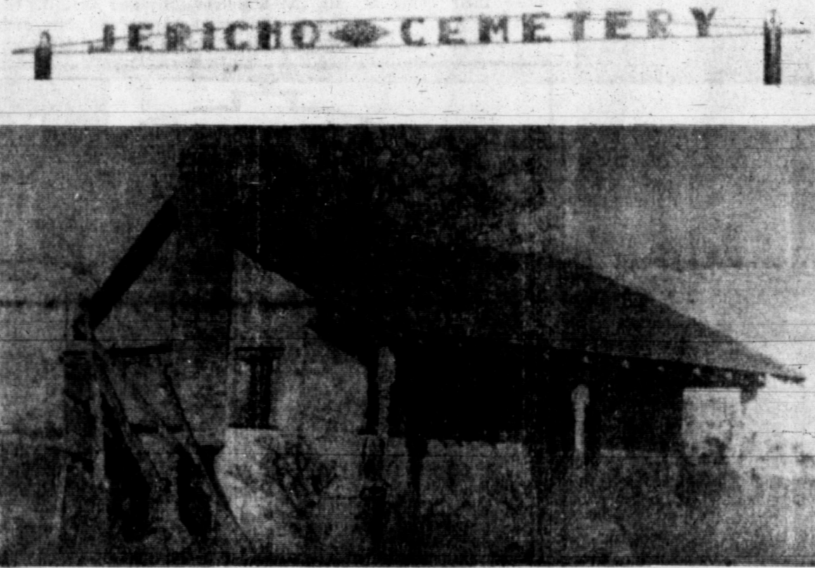
AT REST — Only a few graves were dug in the large Jericho Cemetery (top). Serant's quarters (above) of the Ashmead residence, which burned many years ago, still stand.
