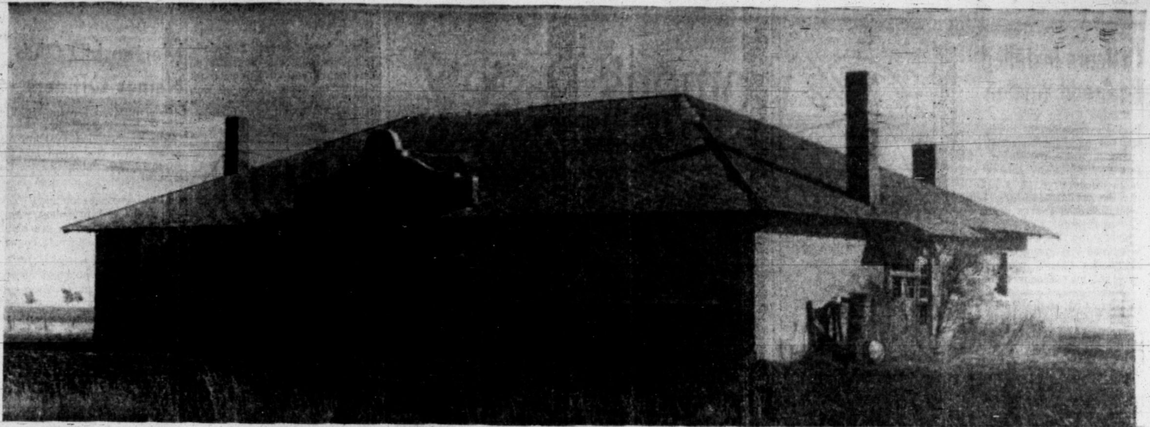
LANDMARK — The most dominant building still remaining at Jericho is the school. Although the sturdy brick structure still stands out strongly against the horizon, the plowed land that surrounds it indicates that the Jericho epic is almost forgotten.
