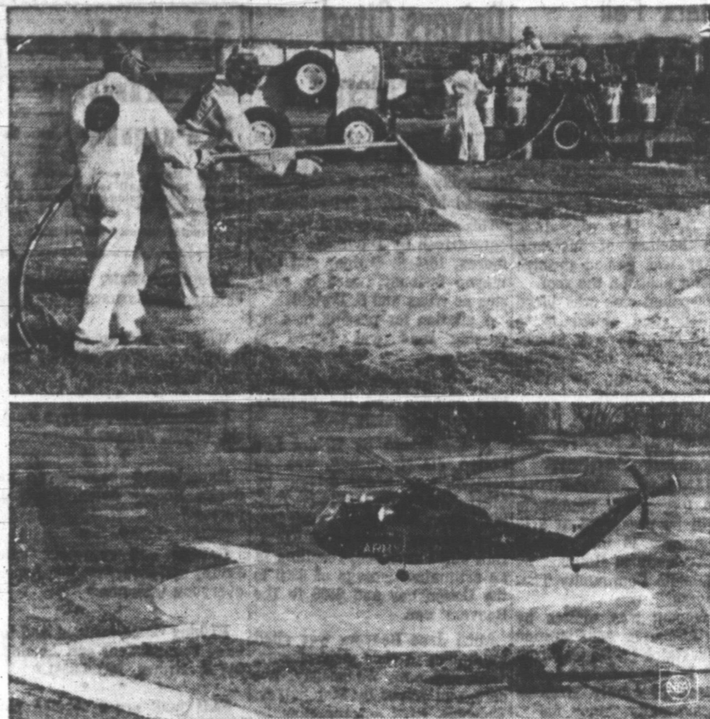
JIFFY LANDING SITE for helicopters and vertical takeoff aircraft is achieved with a new quick-drying polyester resin spray. Above, the mixture is quickly sprayed over a fibreglass mat, hardening in a few minutes to form a pad capable of supporting a landing aircraft, bottom. The technique is being tested in Viet Nam. It can also be used for weatherproof surfacing for ammunition supplies and sandbag emplacements.
