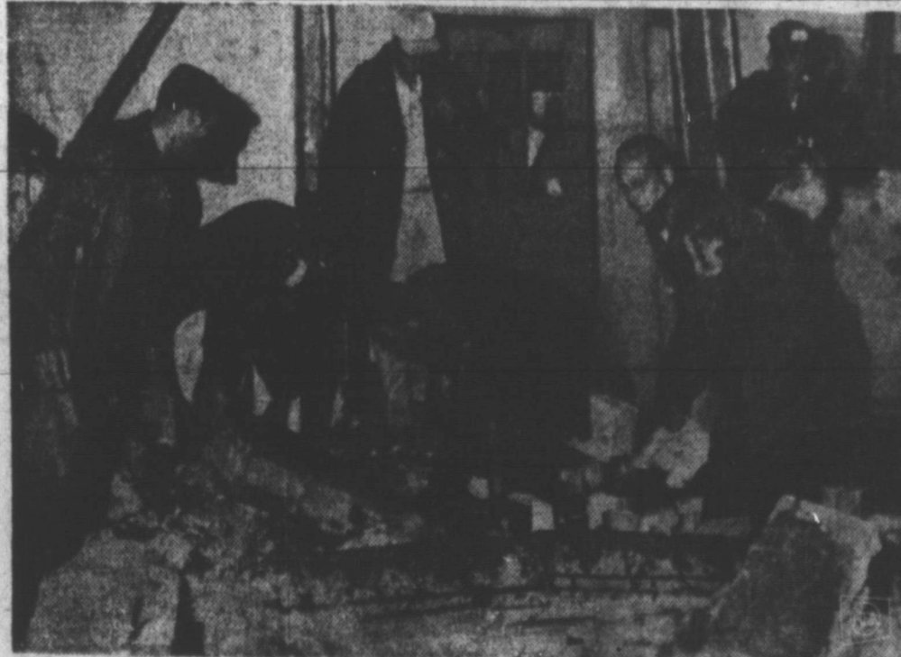
SEARCHING FOR SURVIVORS, firemen dig through the wreckage of the Church of God in Christ at Plainview. An explosion ripped through the Negro church at the start of a week-long meeting of church members from throughout West Texas, killing a Pampa woman and injuring 41 others.
