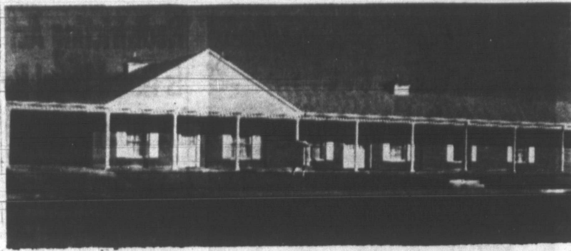
CARMICHAEL-WHITLEY BUILDING — The new home of Carmichael-Whitley Funeral Directors, 600 N. Ward, features a white-trimmed, red brick, colonial architecture.
