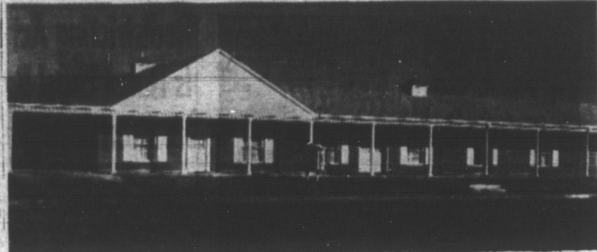
CARMICHAEL-WHITLEY BUILDING — The new home of Carmichael-Whitley Funeral Directors, 600 N. Ward, features a white-trimmed, red brick, colonial architecture.
