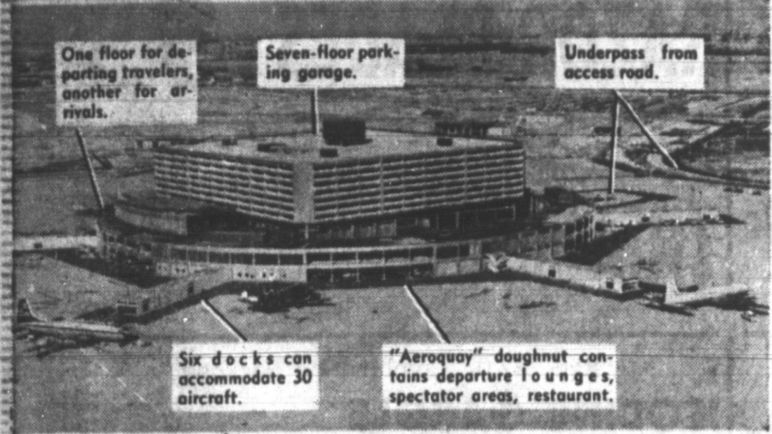
Toronto's air terminal is "in the round." All sides of it can be used because vehicles use a tunnel to approach it. Garage can handle 2,400 cars.
