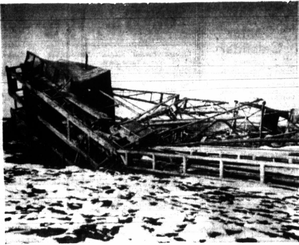
KEERUNCH! — An estimated $15,000 to $20,000 damage was suffered when this drill rig collapsed this past week at Below Lease No. 2 in Wheeler County. The rig, owned by Cantrell and Hoyer Drilling, of Pampa had just started operations the morning of the accident and was at 350 feet when it slowly heeled over, stood at 45 degrees for almost an hour and then collapsed to the ground. A wash-out was believed to be the cause of the accident. The rig was starting a 2,450-foot probe for oil.
