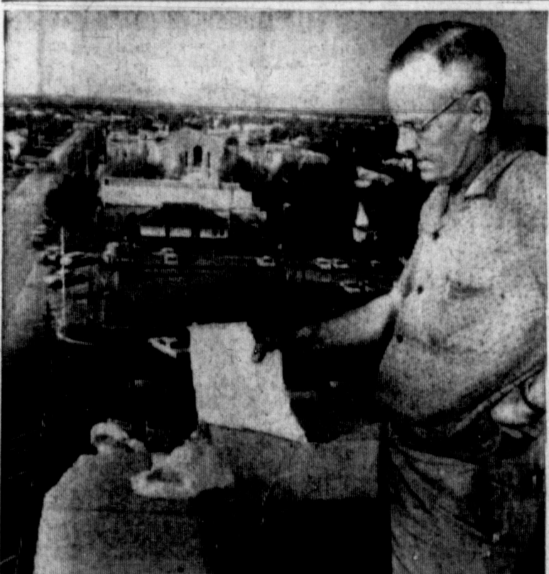
LIGHTNING STRIKES HUGHES BUILDING — Fred Weeks, building superintendent, shows chunks of the structure knocked off during a mid-morning thunderstorm. Weeks had been on the roof shortly before the bolt struck but had climbed down when the storm started. He estimated only nominal damage. The impact was so light that there was no panic in any of the offices.
