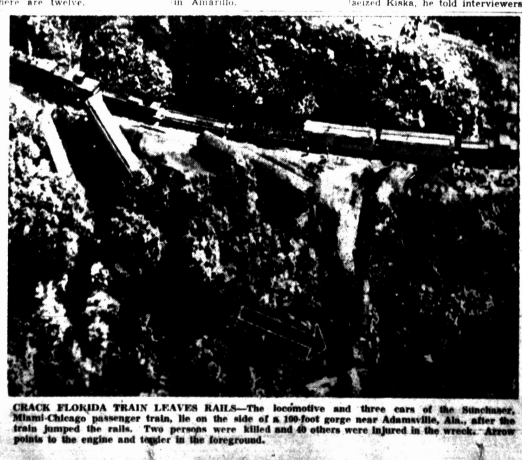
CRACK FLORIDA TRAIN LEAVES RAILS—The locomotive and three cars of the Suncoast, Miami-Chicago passenger train, lie on the side of a 100-foot gorge near Adamsville, Ala., after the train jumped the rails. Two persons were killed and 40 others were injured in the wreck. Arrow points to the engine and tugger in the foreground.
