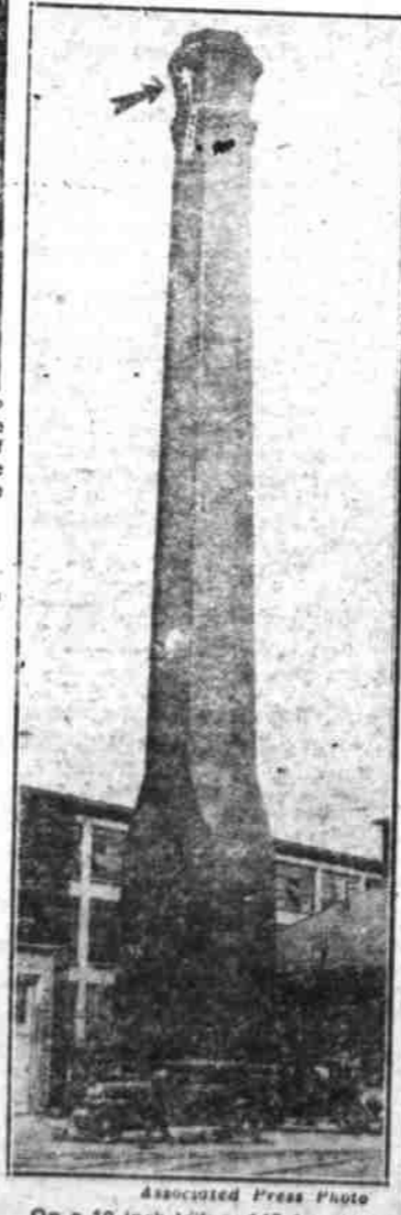
On a 10 inch ledge, 142 feet from the ground, James Kemp, 62-year-old steeplejack, held this precarious perch for two hours in Rochester, N. Y. Bent forward by an outward surge in the stack, he held to a short rope which had broken from a scaffold and sent a fellow worker to death.
