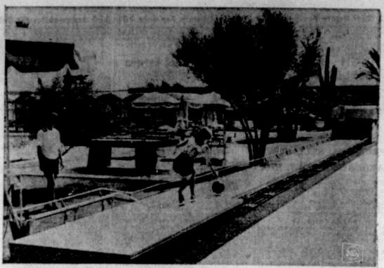
ALLEYS AL FRESCO-Something new in the bowling world is the portable indooroutdoor alley. The alleys are surfaced with hard plywood, feature simplified automatic pinsetters, are constructed in sections and, it is claimed, hold up in almost any weather.
