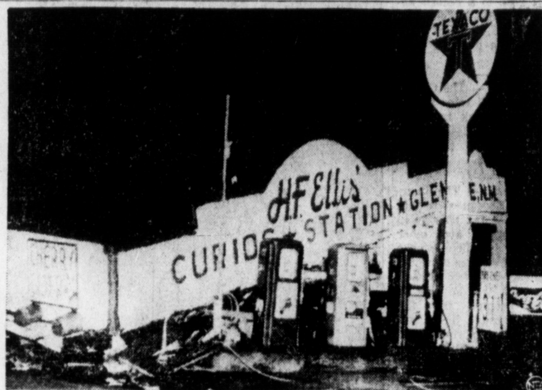
DESTROYED — The store owned by H. E. Ellis at Glencoe, N. M., in the Hondo Valley was destroyed during heavy flooding in the area. Raging floodwaters caused hundreds of thousands of dollars damage, washing buildings, vehicles and equipment downstream.
