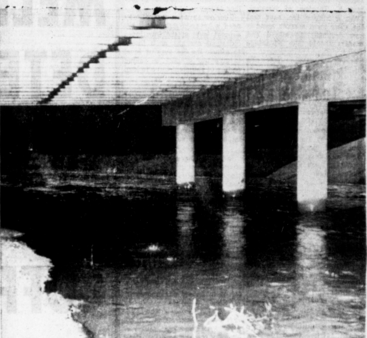
DRAINAGE — It was a wet Tuesday morning in Pampa and the drainage systems showed it. As 1.18 inches fell in Pampa, Red Deer Creek filled with water drained off from the downtown area. The creek is the collecting system for drainage from the downtown district. This morning was one of the few times in recent years that the creek has flowed from bank to bank.
