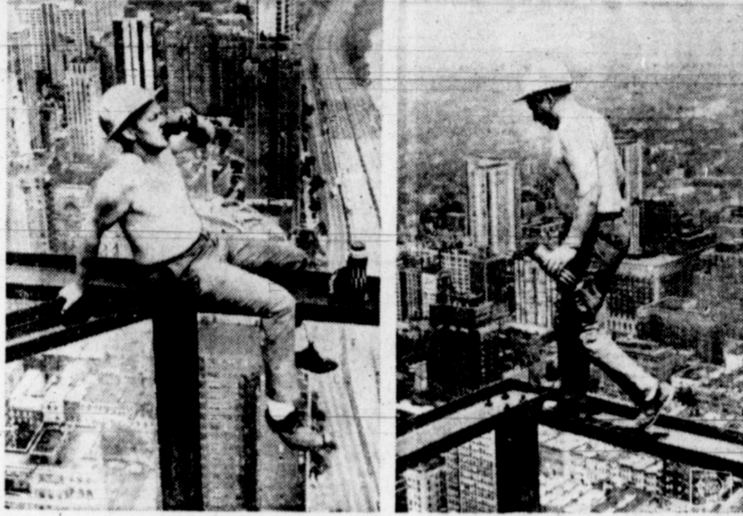
LOFTY LUNCH — In Chicago, concrete superintendent Toroly (Tony) Gusevick gets away from the crowd for a quiet lunch perched 61 stories above street level. Oblivious to all that nothing around him, Gusevick nonchalantly walks back to work after finishing his meal. That's really high living!
