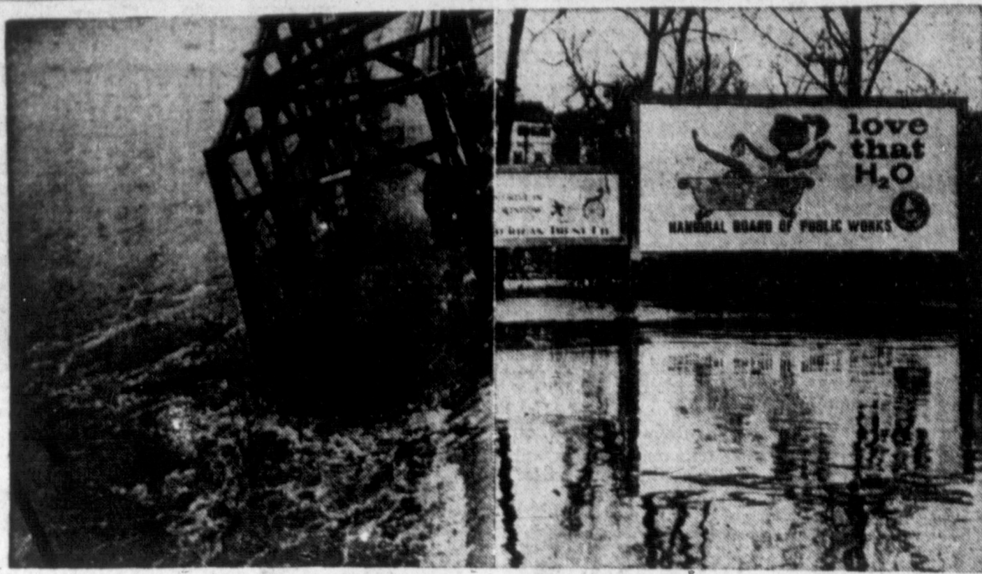
MISSISSIPPI ROLLING ON — Waters of the flooding Mississippi River uprooted the Navy D-land bridge in St. Paul, Minn., and rolled it down-river against a railroad bridge, left. The river reached a record crest of 24 feet above normal in St. Paul. At Hannibal, Mo., the rising waters reach up for a sign that says, "Love That H2O."
