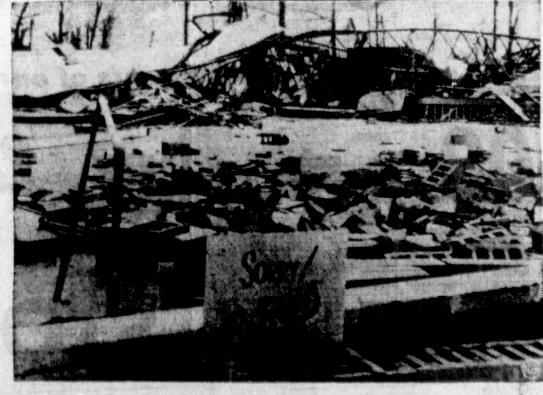
NOT FOR A WHILE — There won't be any dancing at this pavilion in Manitowish, Mich., for a while, at least. A tornado that demolished the pavilion Sunday, leveled most of the buildings in the small southern Michigan community.
