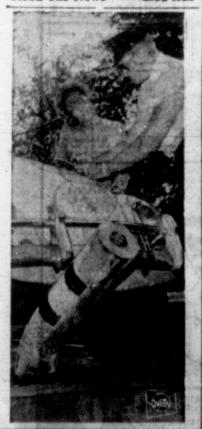
CHECKS BRUISES — About all this woman got when her car collided with the traffic post was a scare and, of course, a ticket. The post is made of rubber, a hollow cylinder seven inches in diameter. Patterned after rubber dock fenders that protect ships, it was developed by an Akron, Ohio, rubber company for highway use.
