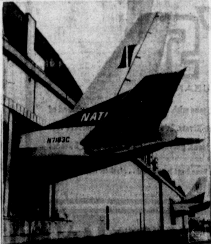
BOAT-IN-THE-CELLAR SWITCH —Visitors to Kennedy Airport, New York, goggle at planes' tail sections protruding from this National Airlines hangar. Special doors with self-adjusting bumpers permit heavy maintenance on the Miami-based jets in a hangar designed for smaller aircraft.
