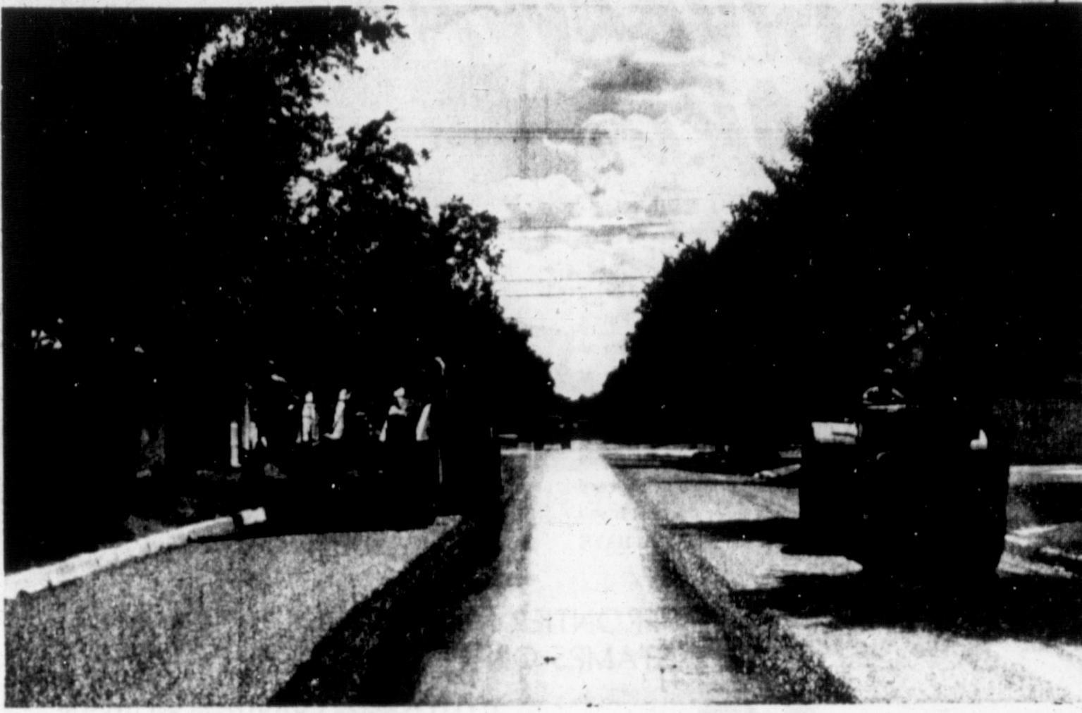
NEW TOP — Two hundred blocks of Pampa's asphalt streets are being covered with a "seal coat" this summer as part of a five-year maintenance program. This is the second year of the program and the 1964 project is about 65 per cent complete. Above, employes of a local construction firm are covering the hot asphalt with selected gravel on the left and rolling the gravel on the right to pack it down. The black strip up the middle of Finch St. is covered with the hot asphalt but still lacks the gravel cover.
