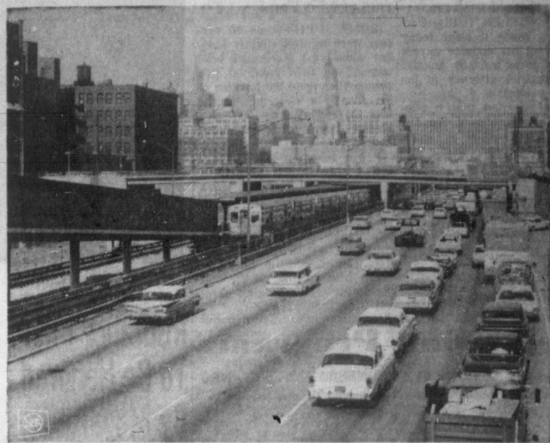
RAIL-RUBBER FREEWAY—Automobiles and rapid transit cars share Chicago's Congress St. Expressway, a major artery in the city's transportation system. The eight-lane highway is split by a rapid transit right-of-way over which thousands of commuters travel each day.
