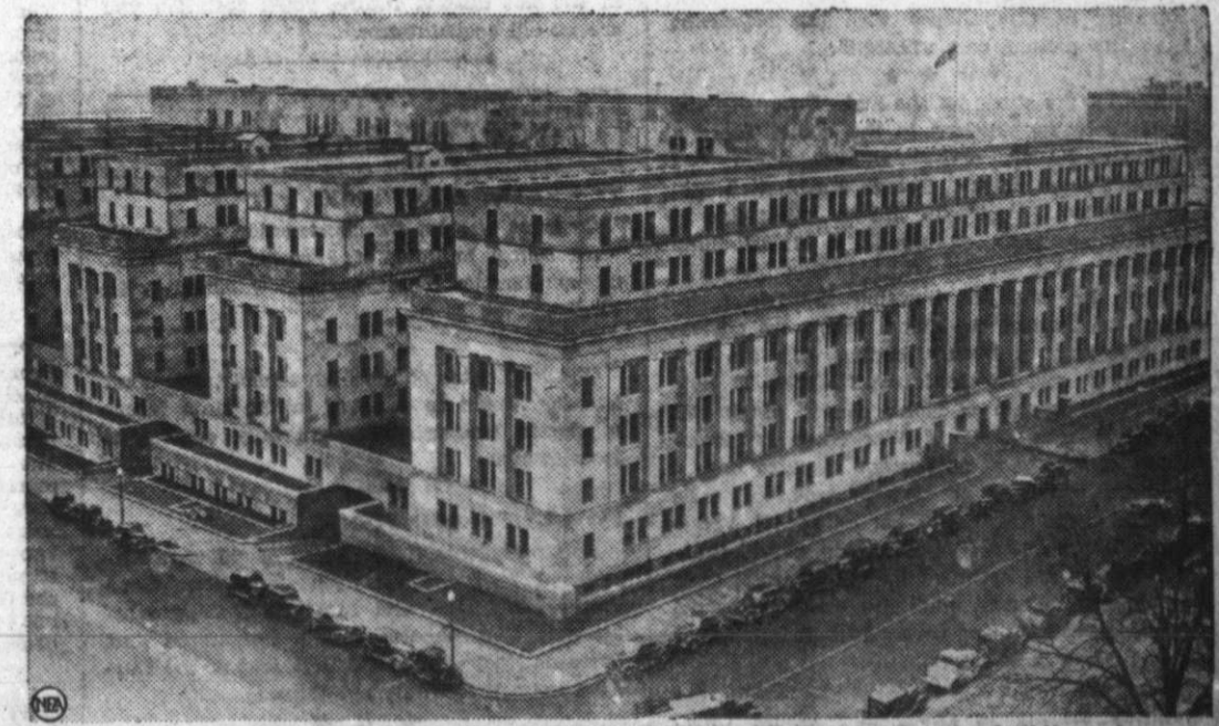
Built to house all the scattered department units under one roof, the new Interior building, above, in Washington, was planned strictly along utilitarian lines, minus frills. It has a wide center wing two blocks long, six block-long wings on each side and will accommodate 3000 workers. It has 1000 clocks, escalators between the first, second and third floors, a 400,000-volume library, auditorium, cafeteria, conference rooms, basement garage and a broadcasting studio. The cost was $13,000,000.
