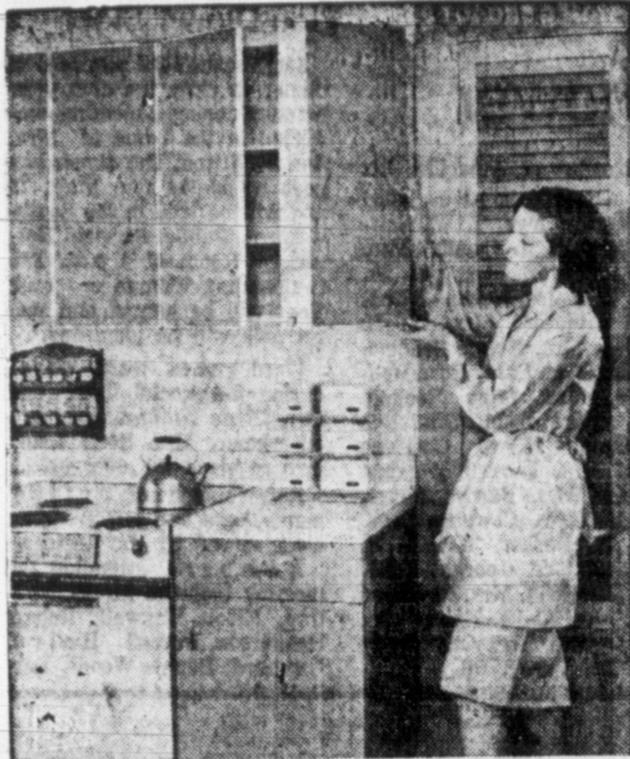
Changing the color scheme in this kitchen is a matter of replacing plastic fronts of enameled steel cabinets. Panels slide into frame.
