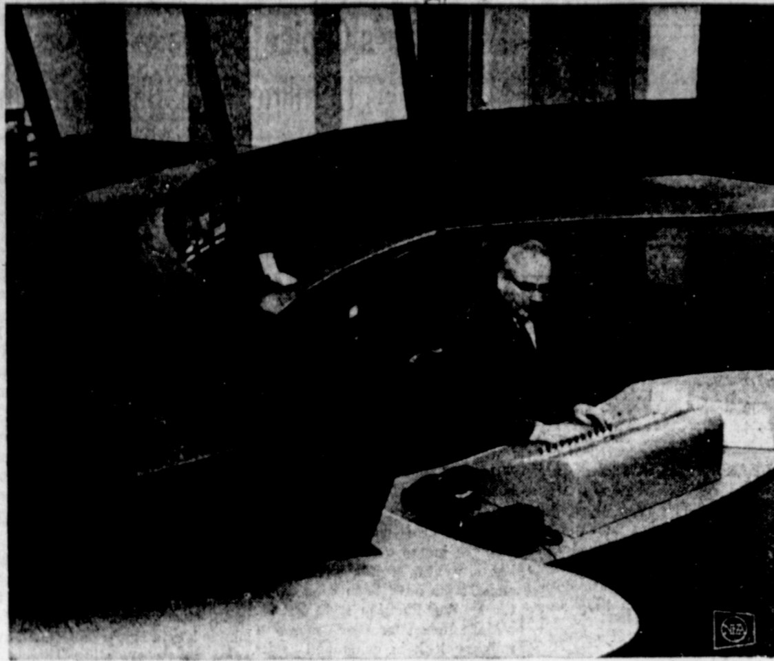
FINGERS ON THE FUTURE —Operator Jim Muirhead makes powerful "music"—hydro-electric power music—on the keys of this space-age-control desk of Hamilton Hydro, Hamilton, Ontario, Canada. Its sweeping design suggesting the control bay of some vast space ship, it provides connections for control of 11 substations, and provision for up to 40 stations total. Electronic devices at the substations perform their remote control functions at touch of a button or a small switch.
