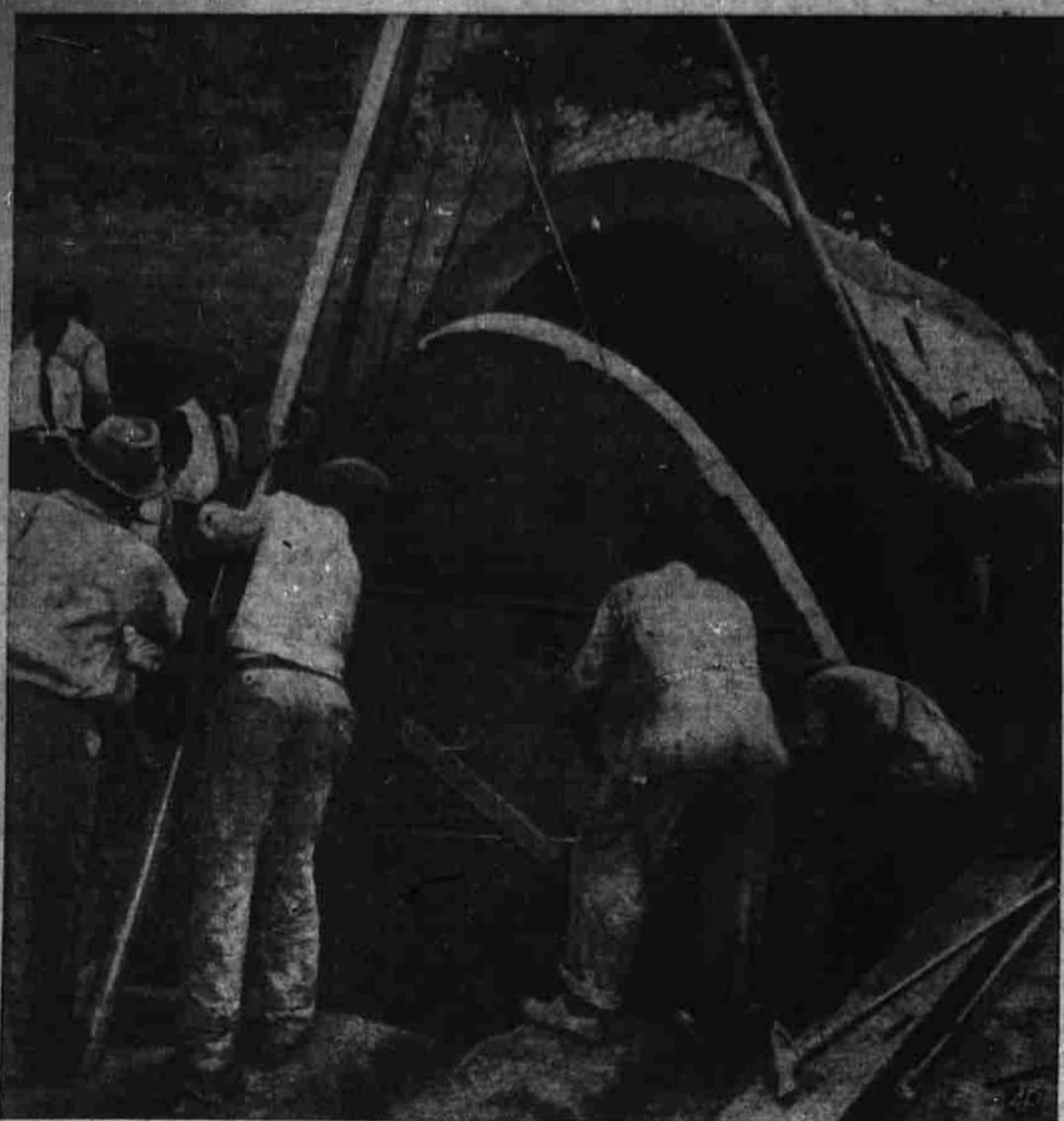
IN FOUR HOURS FLAT this solid concrete bomb-proof shelter was built at Washington, D. C., with military authorities holding a stop-watch on the procedure. The demonstration was to show that bomb-proof fortresses could be built over night. Inventor Karl Billner explains that a vacuum concrete process draws water from the concrete, permitting extra-fast hardening.
