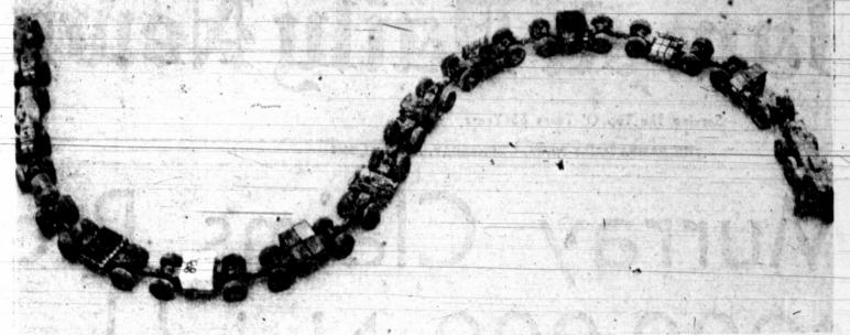
IT GOES 54-HUMMMM-Electric motors-one for each of its 54 giant-tired wheels-powers this experimental Overland Train, snaking its way across the sands at the Army's Yuma Test Station, Yuma, Ariz. Cab, far right,
