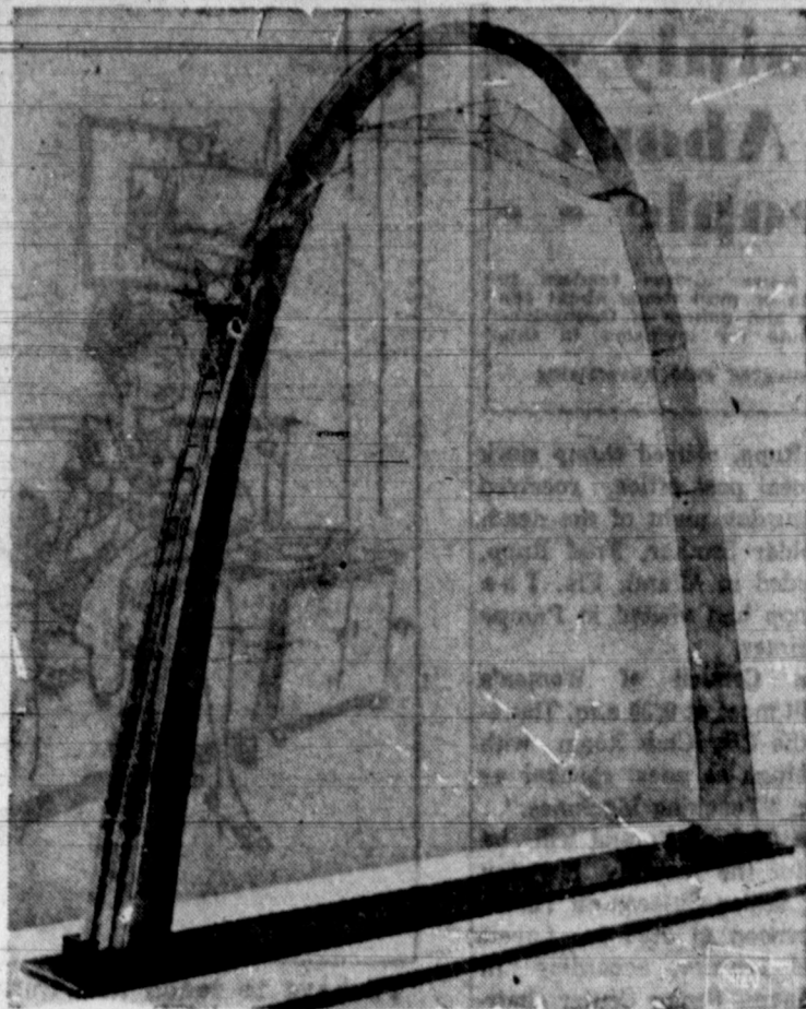
ST. LOUIS ARCH —First 42-ton section of a stainless steel arch that will soar 650 feet above St. Louis, Mo., was completed in Pittsburgh, Pa. It is one of two sections that will form the bases of the towering arch being erected as a monument to America's westward expansion. Model of the St. Louis Arch, right, shows how crane will ride platform up each leg to lift its huge steel sections into place. Tram railway capsule cars, elevators and stairs will be installed in the core of the arch and observation portholes at the top will afford a dramatic view of the city and the Mississippi River. Arch is scheduled for completion in the fall of 1964.
