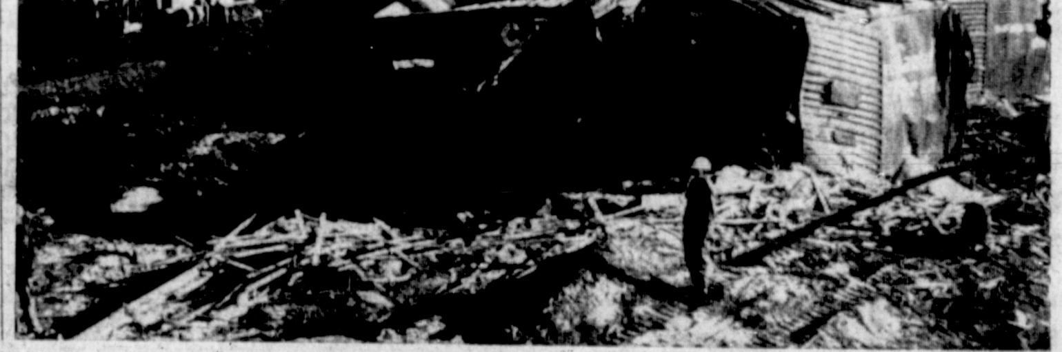
CLEAN UP — Santa Fe railroad workers crews began clean up operations today at the site of a train derailment that happened Friday afternoon a mile and one-quarter east of the Santa Fe depot. Damage to the 23 cars of the 115 car train that derailed, torn up track and pot ash being carried on the train was estimated at $150,000.
