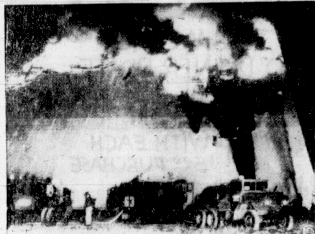
EYE ON SPACE DESTROYER — Flames consume the $30-million "eye on space" radar installation at Elgin AFB, Fla. The new radar system, only one of its type, was used to detect, identify, and track space satellites and missiles. There were no injuries, but a spokesman said the installation was a total loss.
