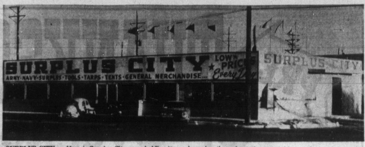
SURPLUS CITY — Here is Surplus City, now holding its "Grand Re-Opening" after having just completed a large remodeling project which gave the firm twice as much floor space as before with a full glass front. There are bargains throughout the store this week and every week at Surplus City, "The Working Man's Friend" in Pampa. (News Photo)
