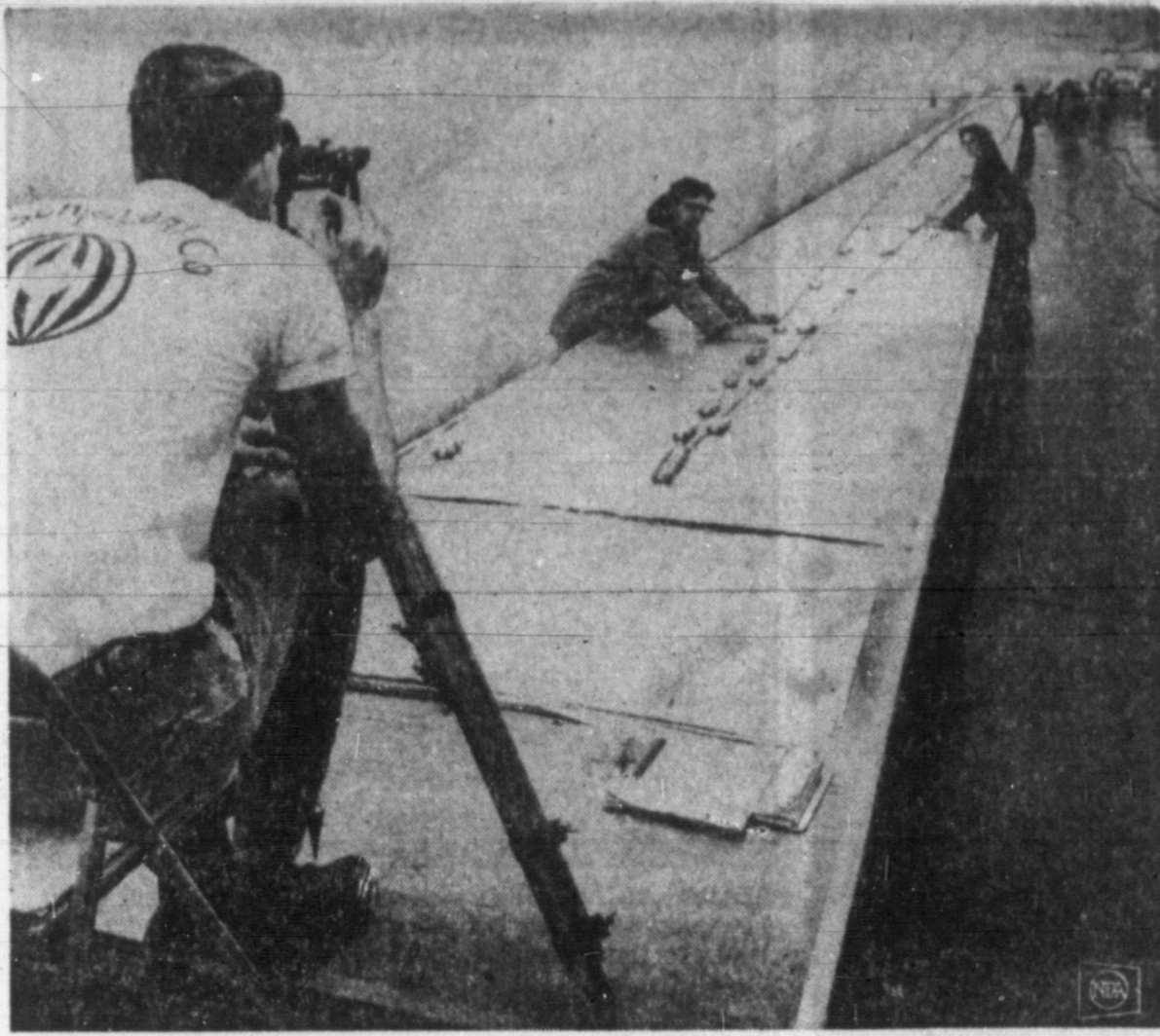
SIC TRANSIT ECHO —A technician uses a surveyor's transit to accurately position 50 layers of material before cutting during the building of a 100-foot-diameter balloon satellite at the G. T. Schjeldahl Co. in Northfield, Minn. Similar to Echo I, which was launched in August 1960, the metal-coated plastic "sateloon" will weigh 125 pounds when fully inflated. Orbiting 1,000 miles in space, the balloon will act as an electronic mirror, reflecting radio, radar and television signals and thereby increase their ranges.
