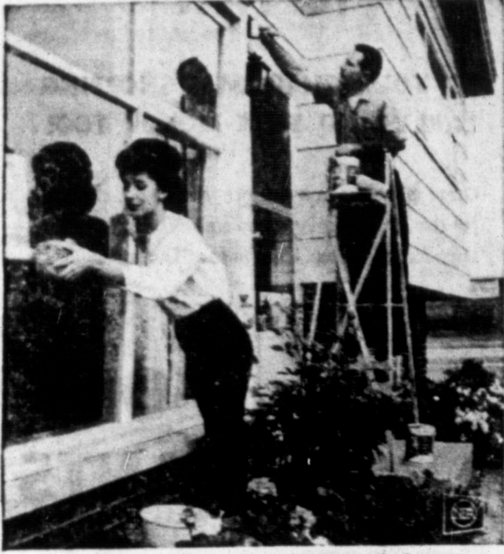
First comes the cleaning and primer coat as the home team goes to work with latex paint.
