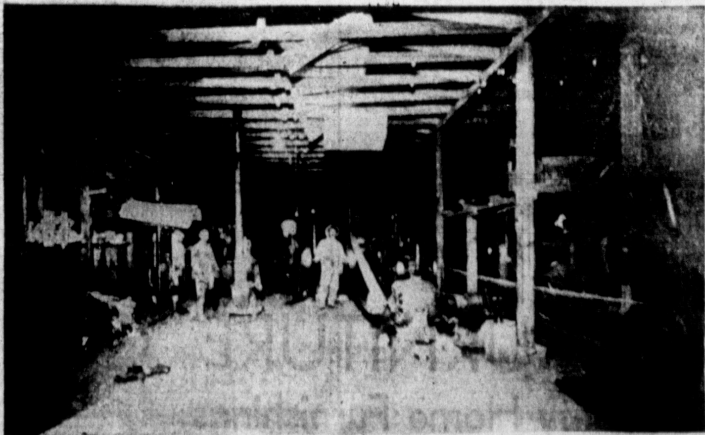
FIRST LIGHT PLANT — Pampa's first light plant was in operation in 1916. The plant was housed in the Davis Warehouse, located on W. Foster Street. Shown here is the interior of the plant.
