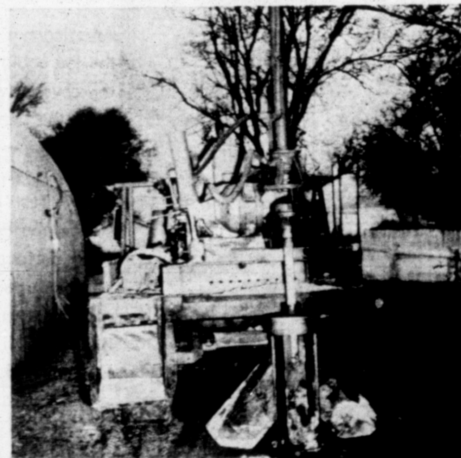
Pictured above — Pier hole digging... running a shaft 18-20 inches and fanning out six feet at the bottom... averts extra work in forming concrete foundation preparations. We have five pier hole drillers available to serve the Top O' Texas area.
