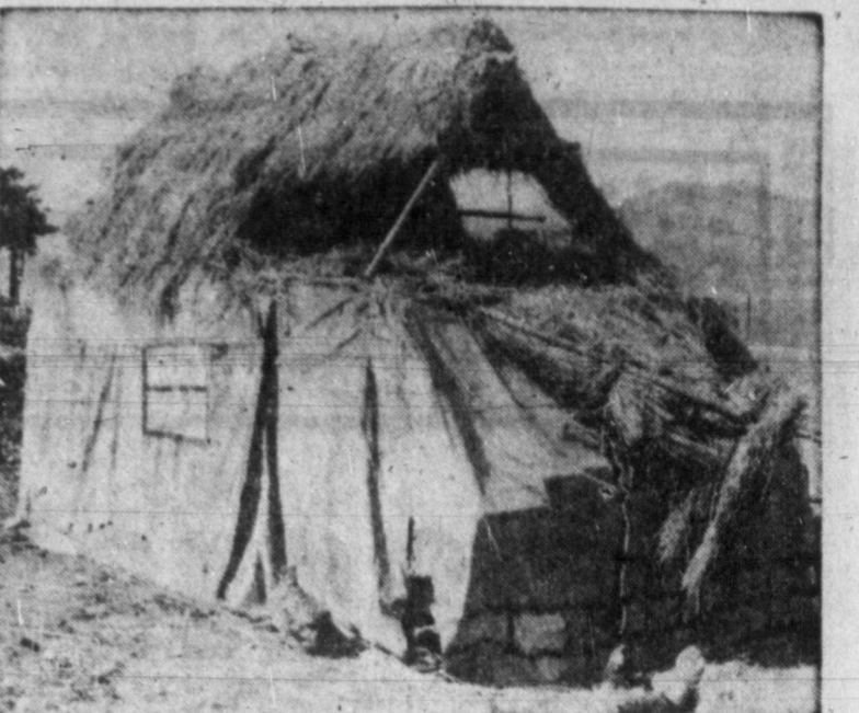
FOOLS 'EM—Little grass-thatched shack in a Korean village is a camouflage project of the U.S. 1st Cavalry Division. The chickens pecking along straw-littered ground are the finishing touch to the hidden armored personnel carrier. "Shack" is shown with portion of roof lowered to permit clear field of fire for a turret-mounted .50 caliber weapon.
