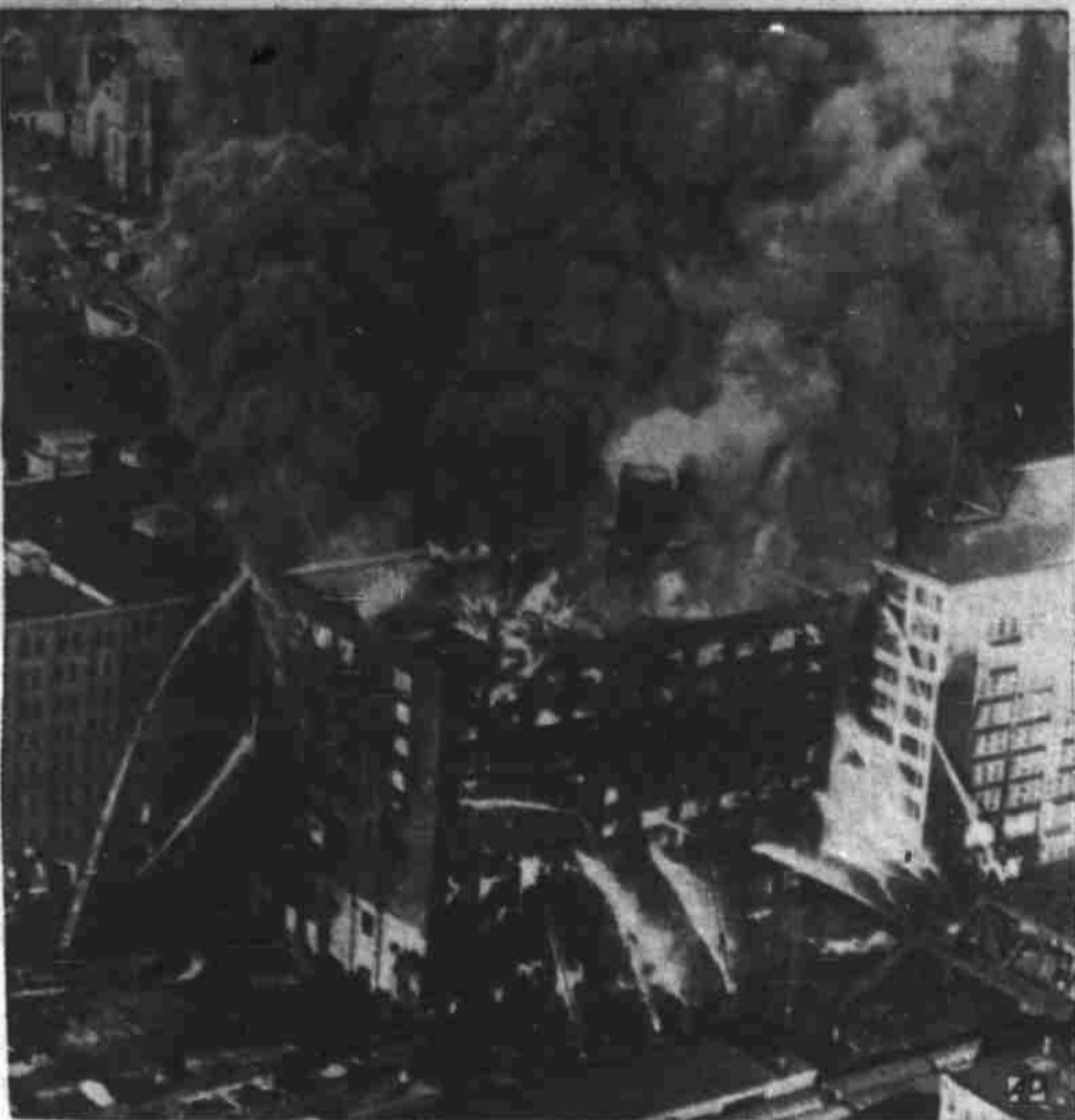
Fire Wrecks Warehouse
