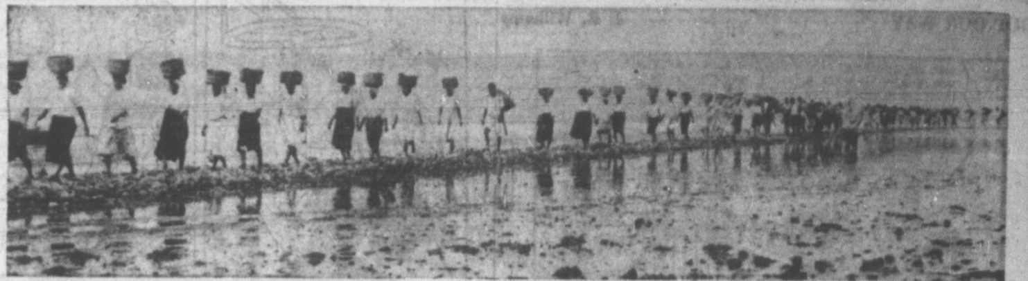
HUMAN MACHINE—Men and women haul dirt for soil reclamation project along the Yellow Sea coast near Chang-hung, South Korea, where machinery is scarce, in an effort to gain new farm lands to feed an increasing population.
